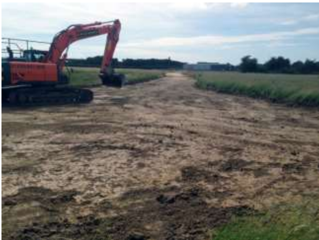
Plate 24: Showing overburden removal in area BSF-WB-15. Looking west.
